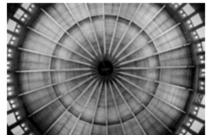
DuSable Museum Roundhouse original timber dome ceiling. DuSable converted a former horse stable to exhibition space. Duane Savage.
