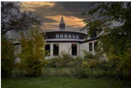
DuSable Museum Roundhouse, a former horse stable converted to exhibit space. Designed by Daniel H. Burnham of timber and limestone in 1800's. Diane Halle
